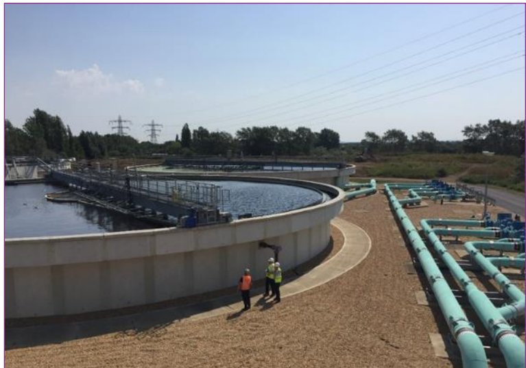
Figure 2-9: Existing Cambridge Final Settlement Tanks
