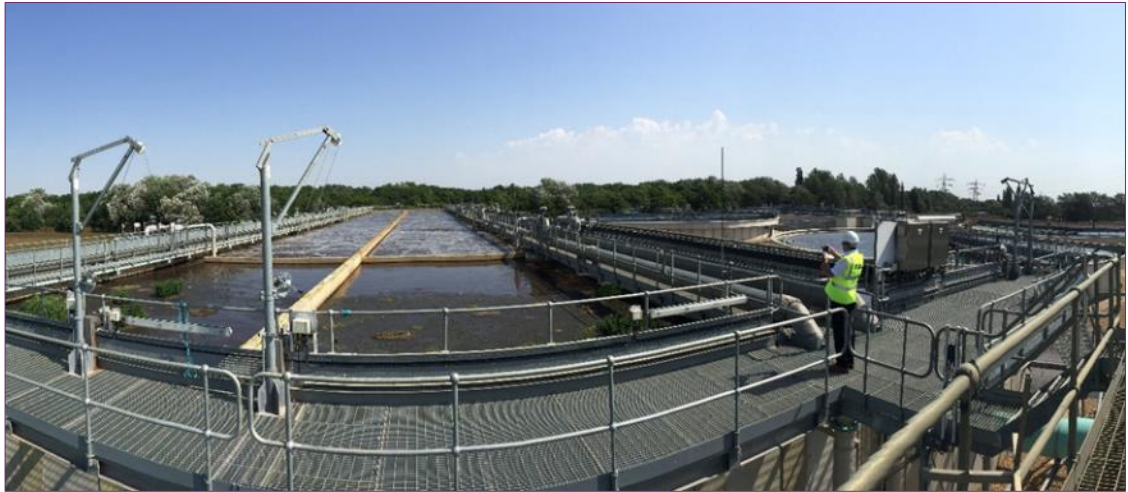
Figure 2-8: Existing Cambridge Activated Sludge Process
