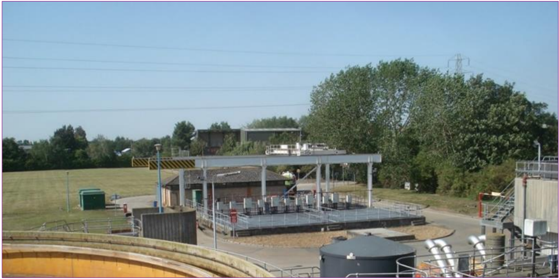
Figure 2-4: Current Terminal Pumping Station at the Existing Cambridge WWTP
