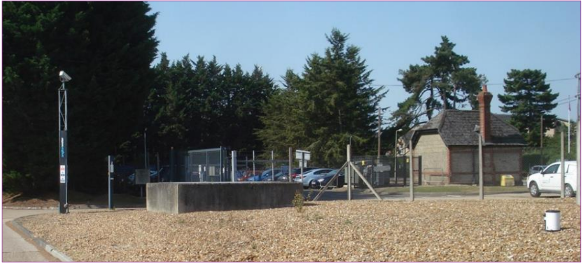
Figure 2-18: Example fencing and CCTV camera
