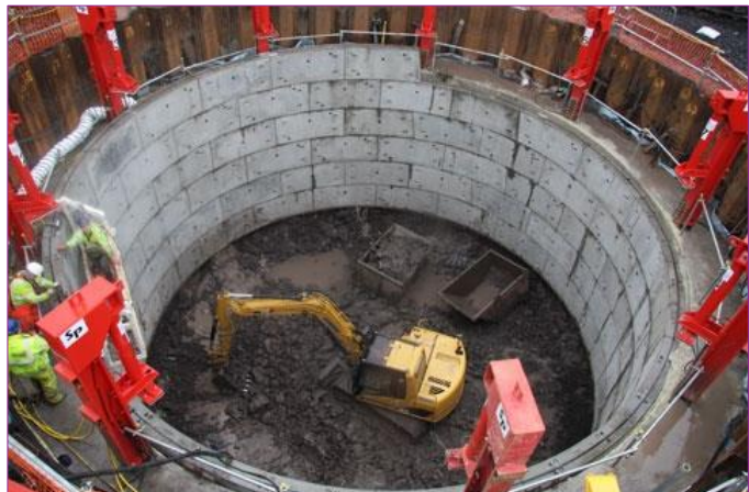
Figure 2-5: Example shaft construction
